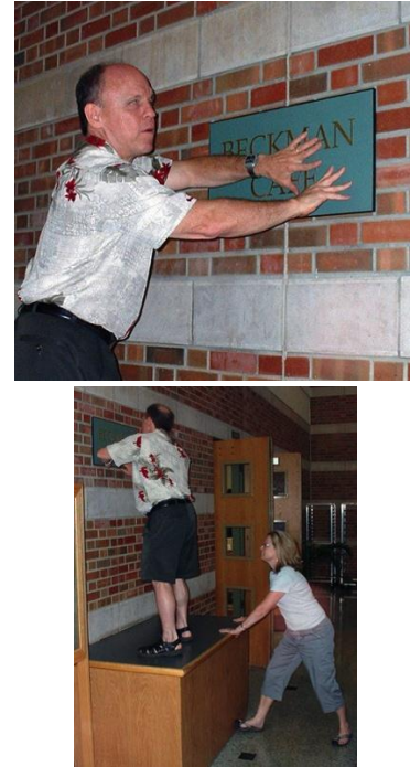
Figure 3: Extreme functional failure: Braille signage meets regulatory requirements but not user needs
