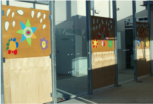
Playground Panels - internal view during installation.
